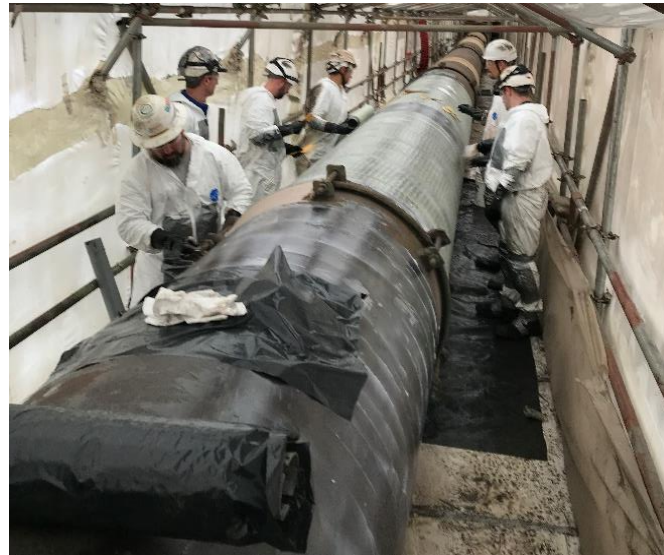
Step 2: Installation of GFRP/CFRP System
